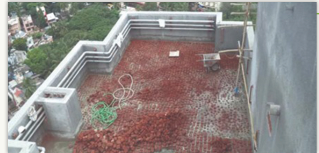
Brickbat Coba Water proofing For Terrace
