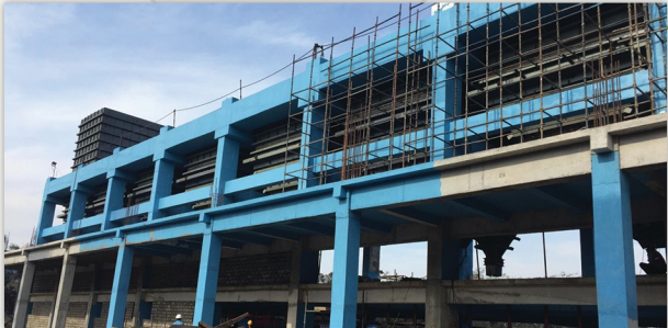
Anti Carbonation Paint @ Rain Cll Carbon Ltd.
