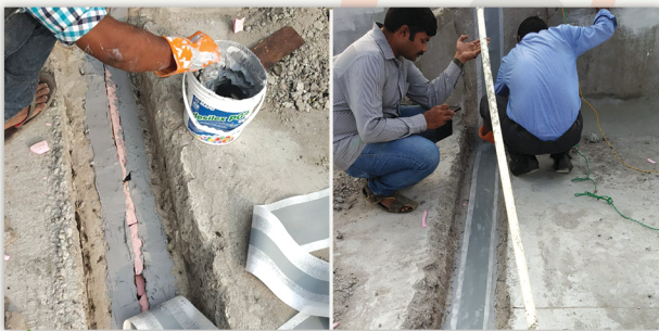
Expansion joint treatment @ Mk gold coast
