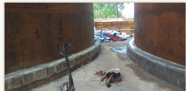
Non -Shrink Grout Application work under oil tanks @ kakinada Gemini Edibles and Fats india Pvt.LTD.
