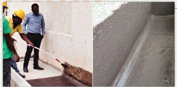
PU Waterproofing @ Mk Gold coast
