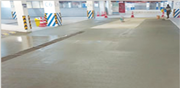
SRMT- Anti skid epoxy Flooring work
