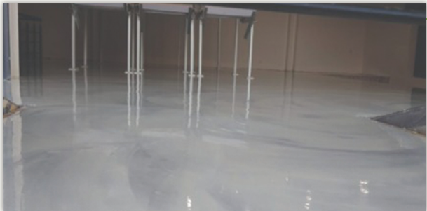
Epoxy Flooring ( 4mm Thickness) at Loading Bay @ Sanken
