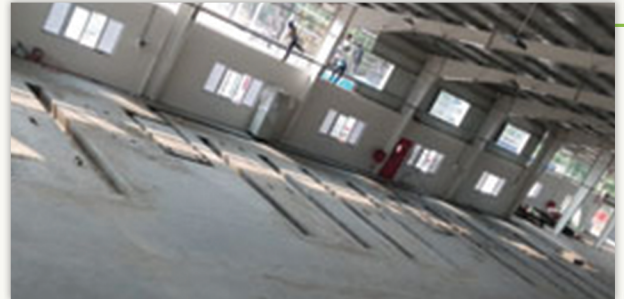
Machine Foundation Non- Shrink Grout @ Jayaa Construction
